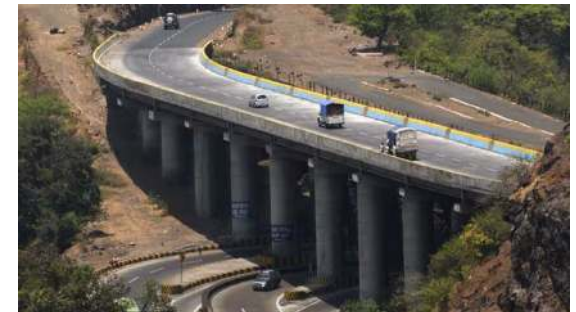
MUMBAI - PUNE EXPRESS WAY
